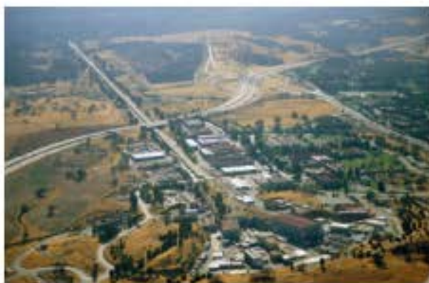
FIGURE 9.3.2 Aerial photograph of the Stanford Linear Accelerator Center, California, showing the 3.2 km linear accelerator housed in the world's longest building. Particles are accelerated from the top left to the detectors in the foreground.
