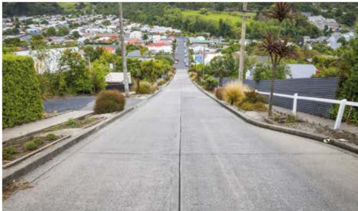
FIGURE 2.1.1 The steepest residential street in the world. Its upper level is surfaced in concrete—bitumen would flow down the slope in warmer temperatures.
