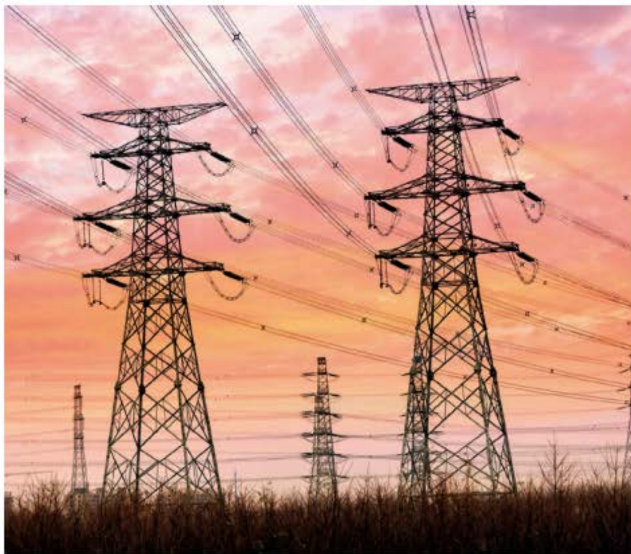
FIGURE 5.1.19 Each one of the current-carrying wires running between the transmission towers will generate a magnetic field around it, as long as a current is flowing.
