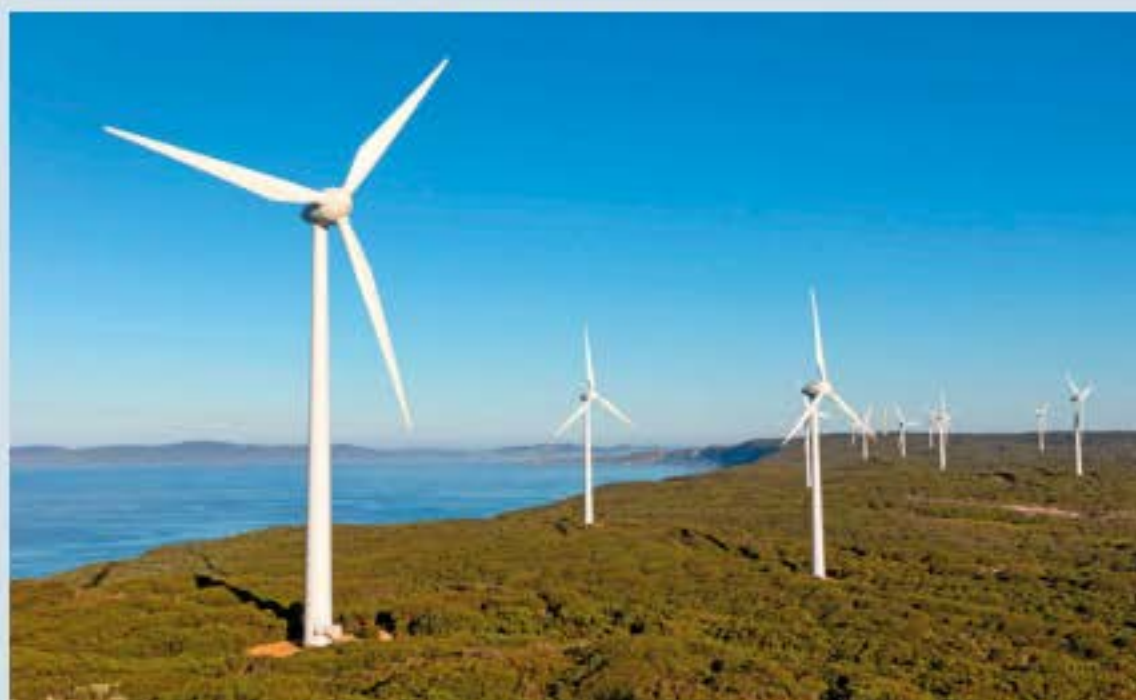
FIGURE 2.4.4 The tips of these wind-generator blades are travelling in circular paths at speeds of around 290 \text{ km h}^{-1} .
