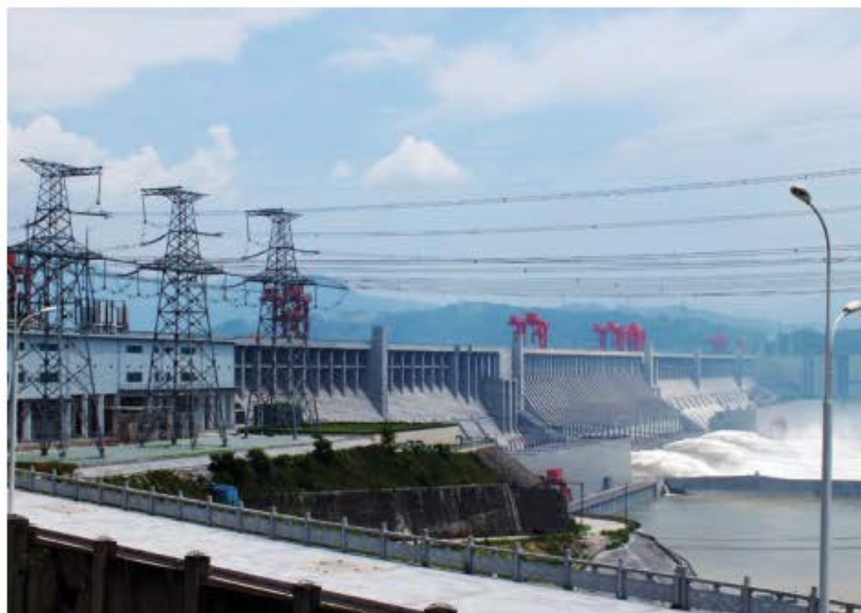
FIGURE 6.4.13 At the Three Gorges Dam in China, engineers are considering the use of DC transmission at higher voltages than is possible with AC to further reduce transmission losses.
