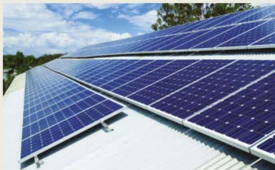
FIGURE 7.4.13 Solar panels are used to convert sunlight into electrical energy using the photoelectric effect.
